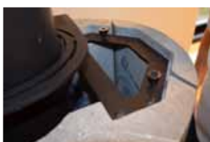
14: Lock the 4 top stones using the accompanying locking brackets. Ensure that the locking brackets have been pressed completely down in the holes in the soapstone.
