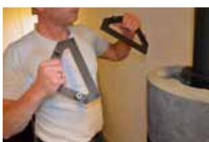
14: Lock the 4 top stones using the accompanying locking brackets. Ensure that the locking brackets have been pressed completely down in the holes in the soapstone.
