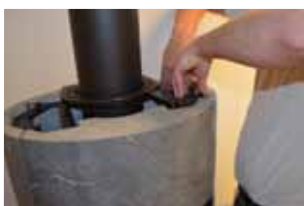
17: Now remove the one locking bracket in the top and carefully remove the side stone.
