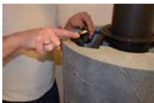
16a: Loosen the side stones one at a time and adjust them in so that they are level with the top stone, then tighten the side stone again.
