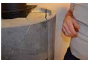
19: Remount the side stone and locking bracket.
