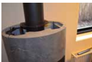
17: Now remove the one locking bracket in the top and carefully remove the side stone.
