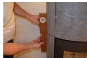
16a: Loosen the side stones one at a time and adjust them in so that they are level with the top stone, then tighten the side stone again.
