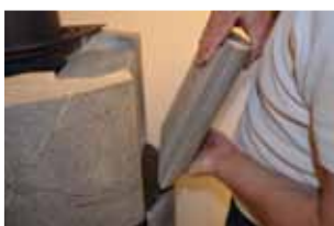
19: Remount the side stone and locking bracket.
