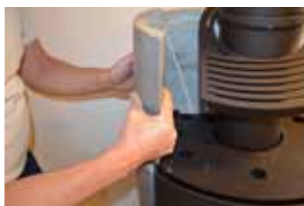
12: Now mount the 2 side stones in the same way as in point 11. BE CAREFUL THAT THE STONES DO NOT FALL DOWN.
