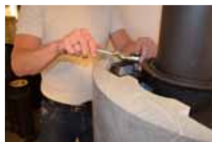
16a: Loosen the side stones one at a time and adjust them in so that they are level with the top stone, then tighten the side stone again.
