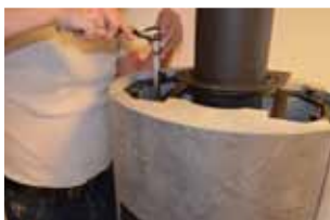
16a: Loosen the side stones one at a time and adjust them in so that they are level with the top stone, then tighten the side stone again.
